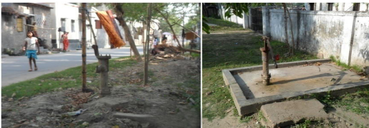
Plate 1: Effect of ground water table depletion at hand tube well, Rajshahi city.
